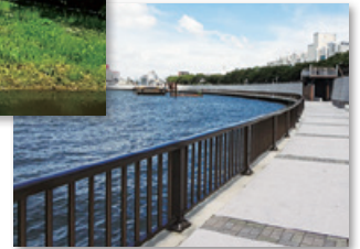
Response to climate change (installation of high-tide defense facilities)
